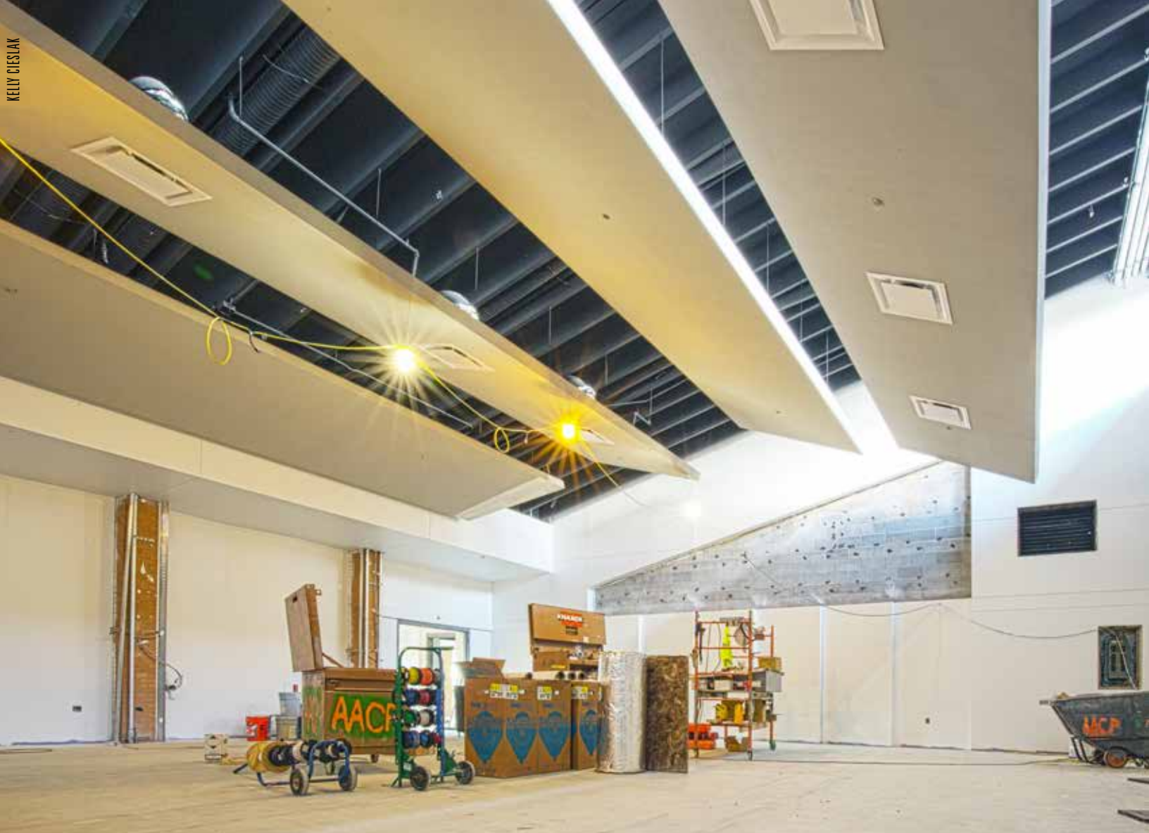
Above: Rehearsal space under construction. Right: Rendering of completed room.
